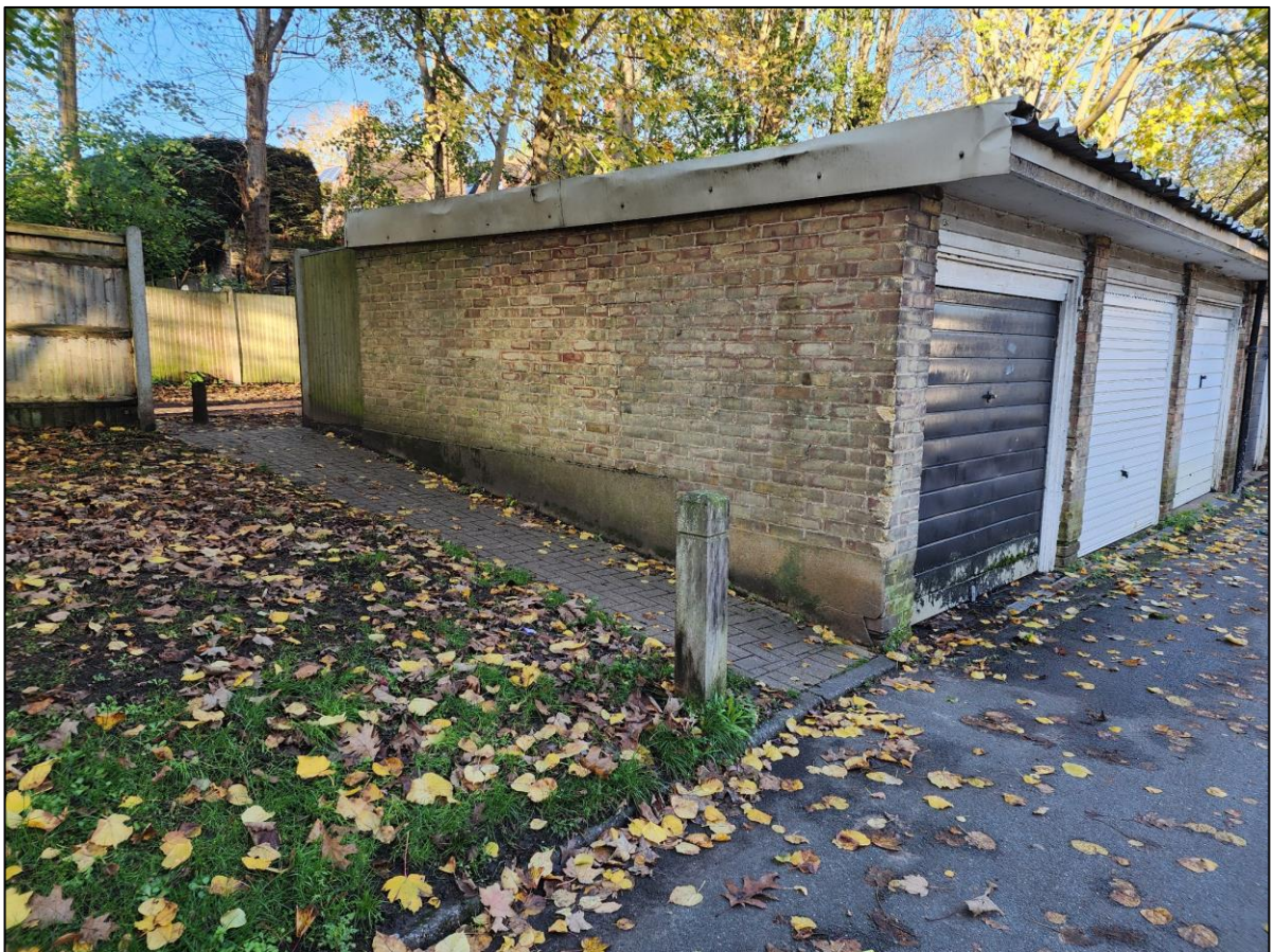
Figure 2.6 Access to Putney Park Lane from Innes Gardens
