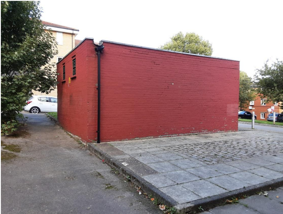
Photograph 5: Substation, building B1
