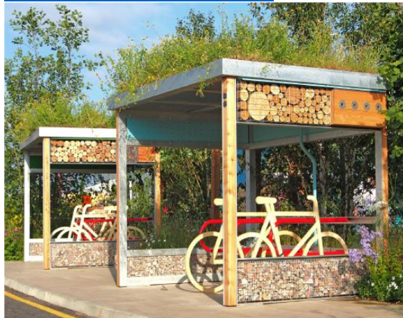
Figure 1. Example of green roofed cycle store http://greenroofshelters.co.uk/
