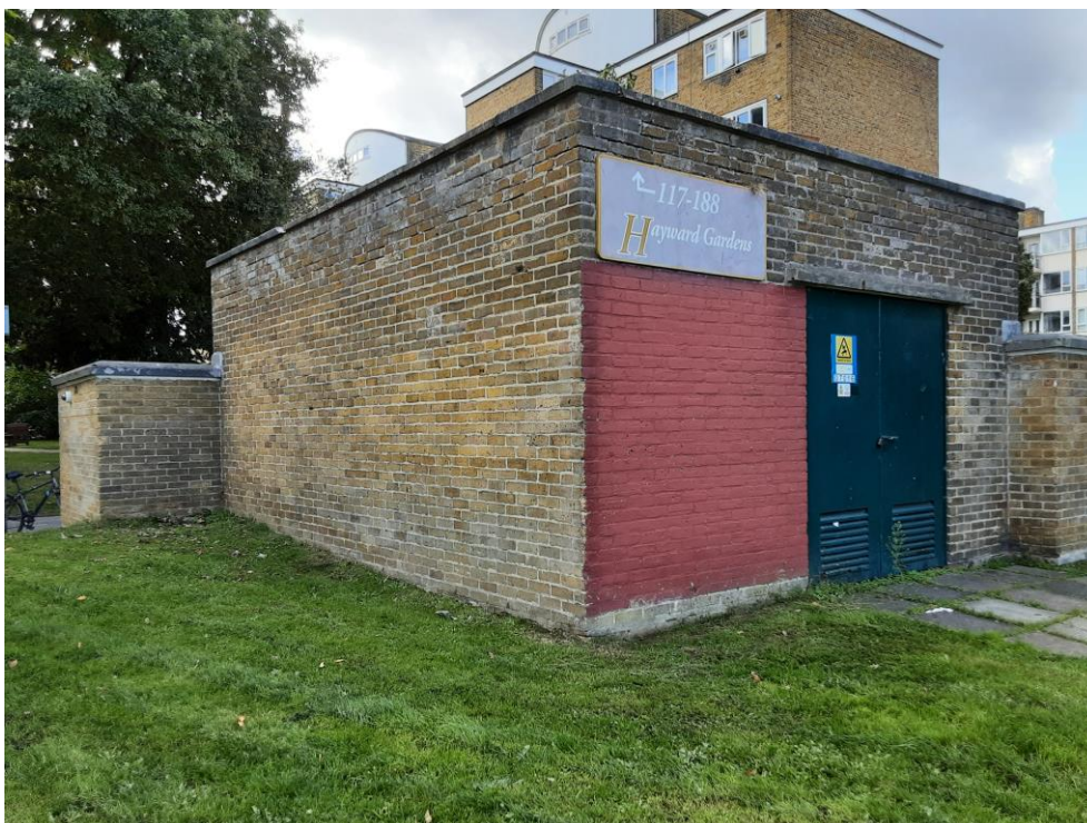
Photograph 3: Substation building (B1) within Site 2
