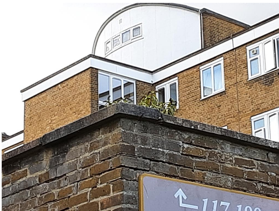
Photograph 5: Butterfly-bush (Invasive species 1, Figure 2) on the roof of B1 within Site 2
