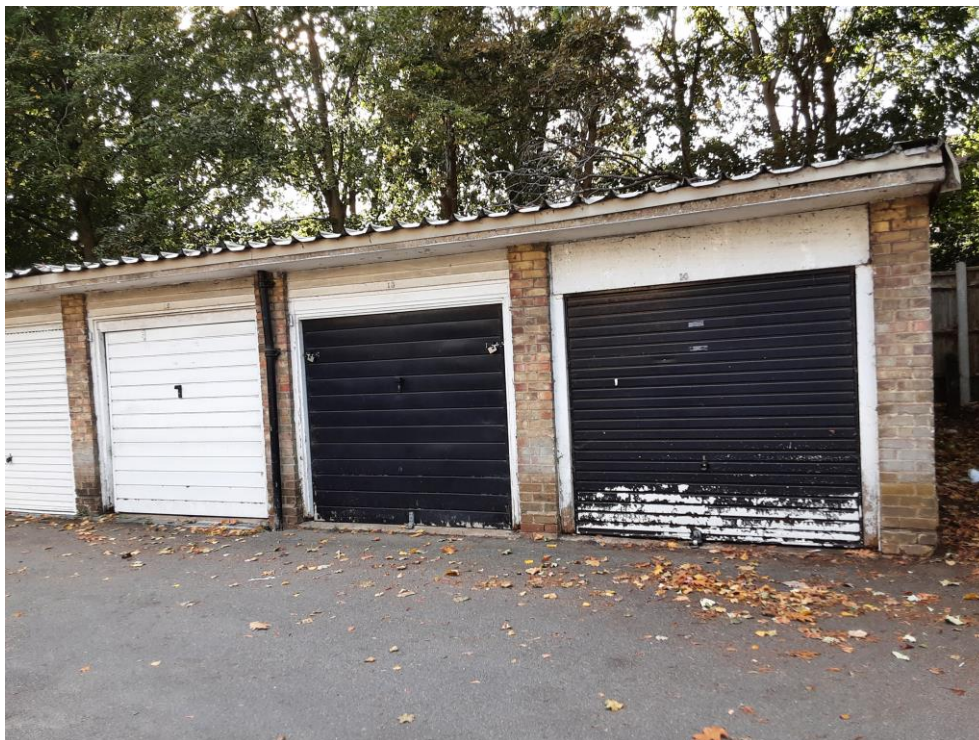
Photograph 9: Building B2 on Site 1
