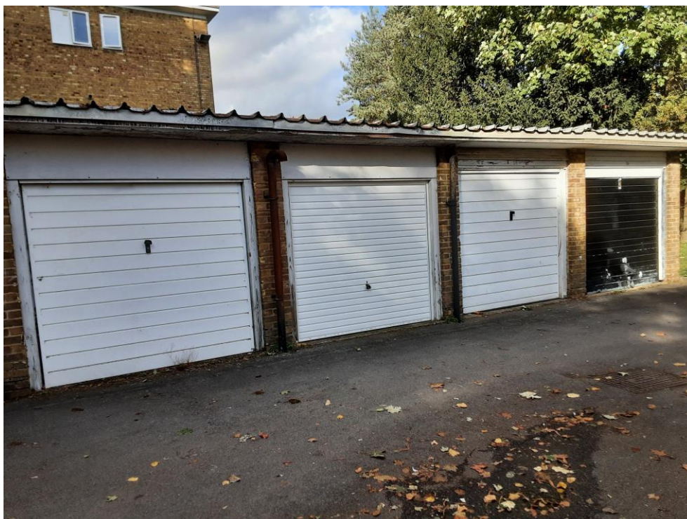
Photograph 3: Building B1 on Site 1
