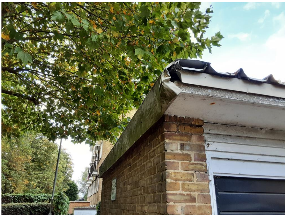
Photograph 5: Access into garage in Site 1
