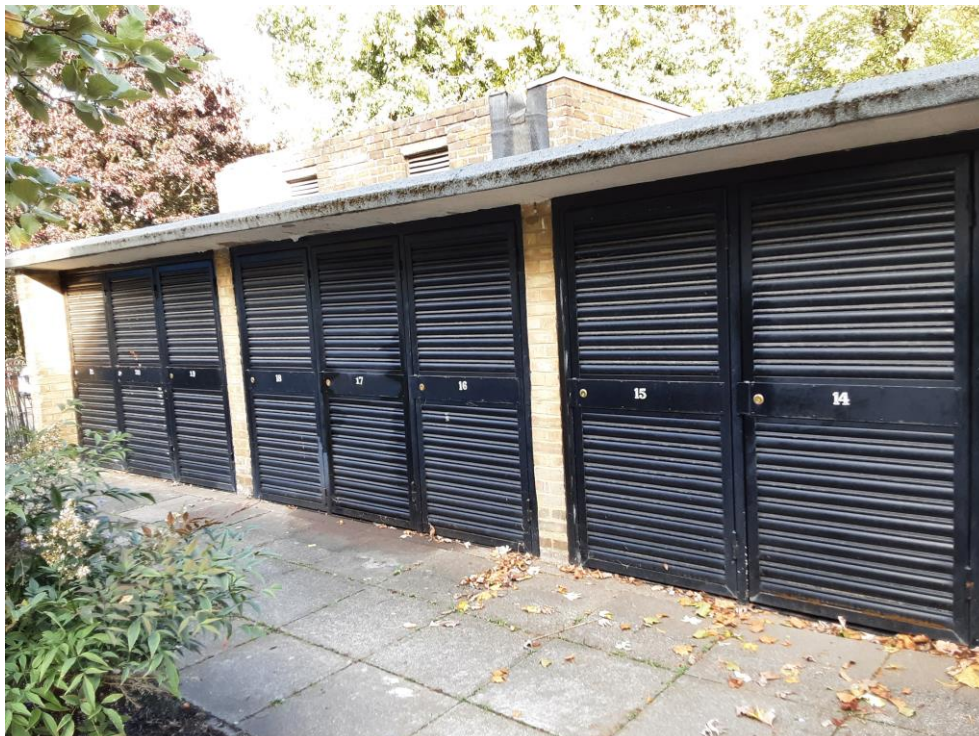
Photograph 4: Storage units in Site 2
